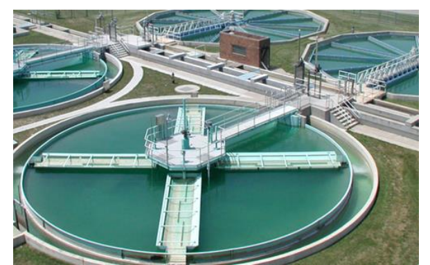
Tertiary Treatment near STP
