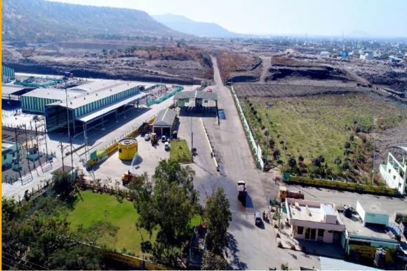
Main Trenching ground/ Landfill site
