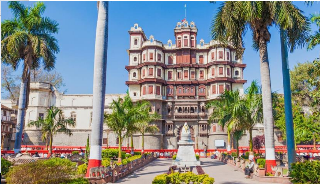
Conservation & Restoration of Rajwada
